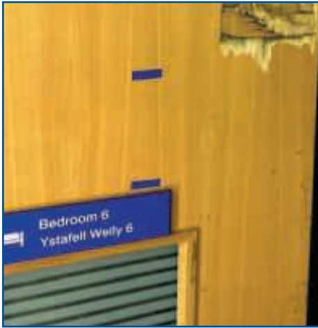
◀ Typical damage caused when a double swing door is forced — Protector in place
